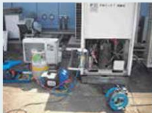
Pump out the current refrigerant in the pipe.
