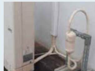
After installation of the device, put thermo-insulator.
