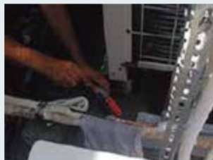
Apply silver welding in order to prevent any gas leakage.
