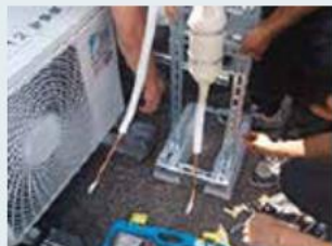
Insert \alpha -ESG between the cutoff pipes.
